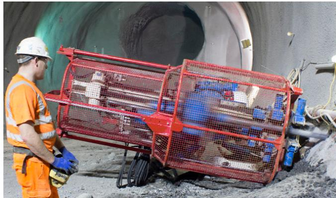
The SM5 is a compact rotary drilling rig that is ideally suited to in-tunnel augering and well drilling, and working in confined conditions such as basements, tunnels and shafts.
